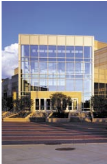
PHOTO COURTESY OF INDIANAPOLIS CONVENTION & VISITORS ASSOCIATION
